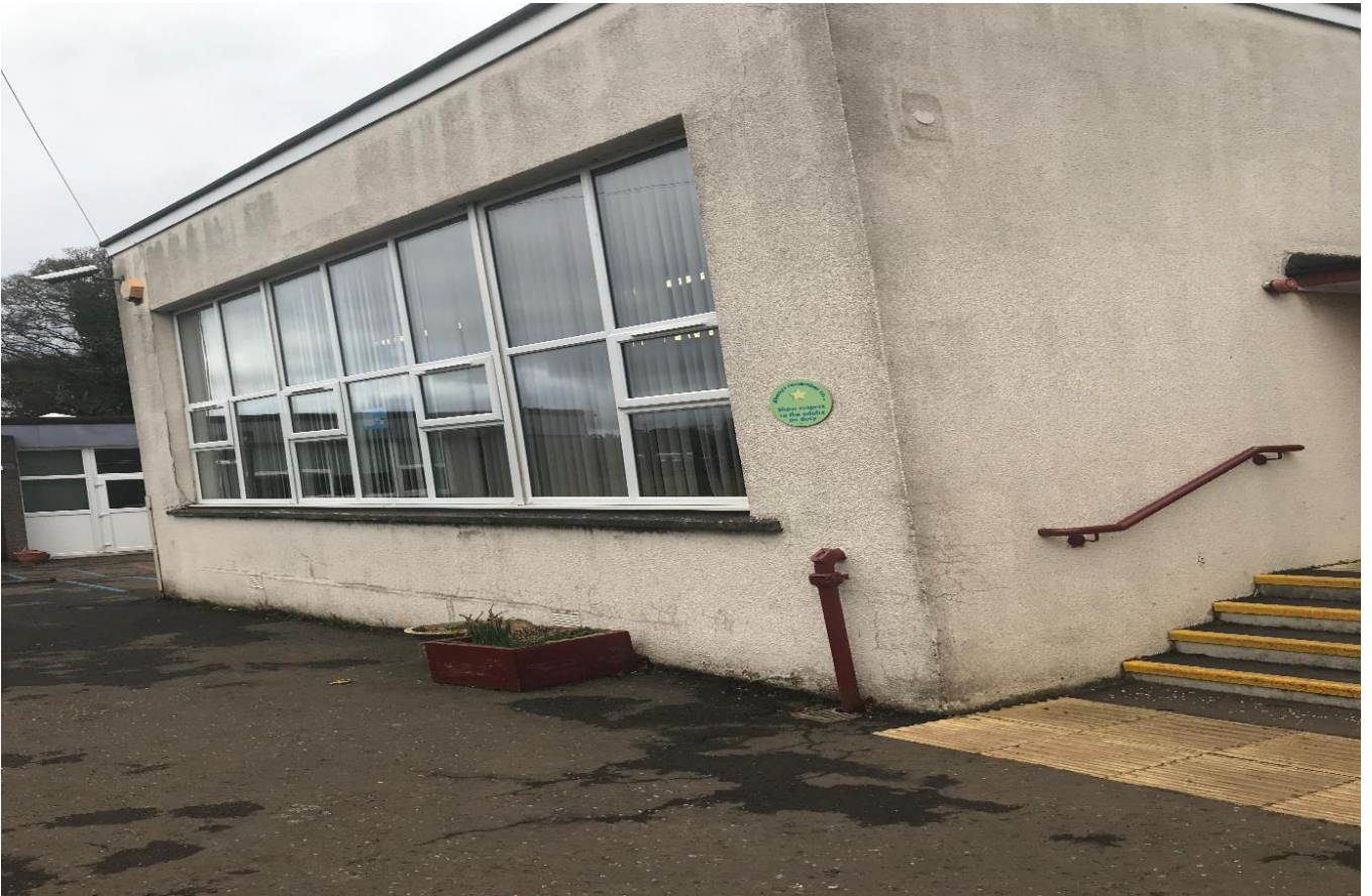
Photograph of External Wall at St. Margarets PS before Enhancements
